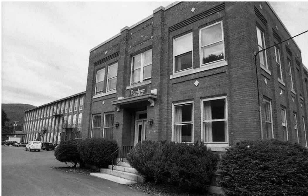
The main entrance of Dunham Brothers at Cotton Mill Hill in Brattleboro. Provided photo
